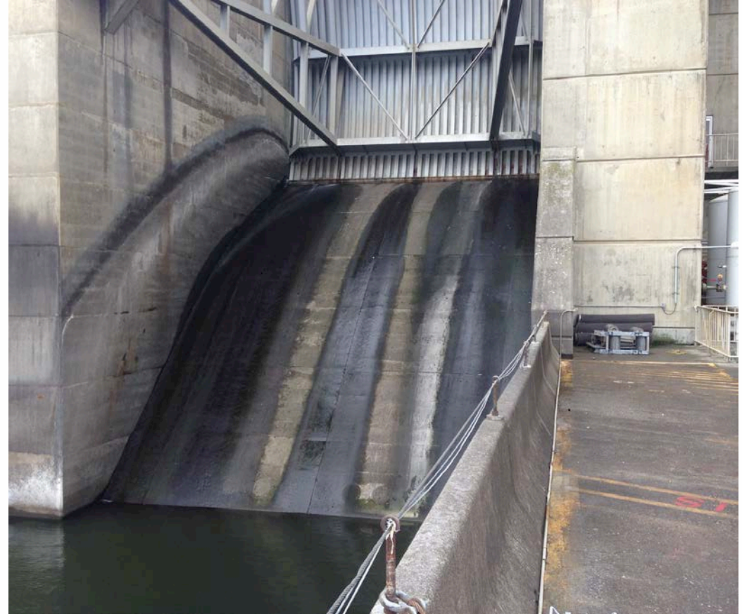
Figure 10. LGR spillbay one, dewatered – Gabriel Brooks, NOAA
