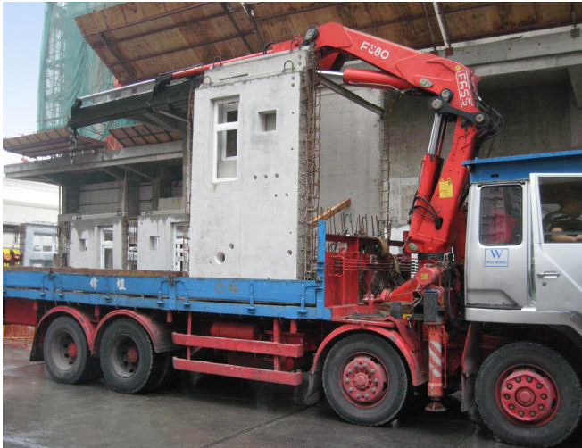
Passive RFID tags embedded in precast concrete facades let contractors track when they are delivered and installed.
