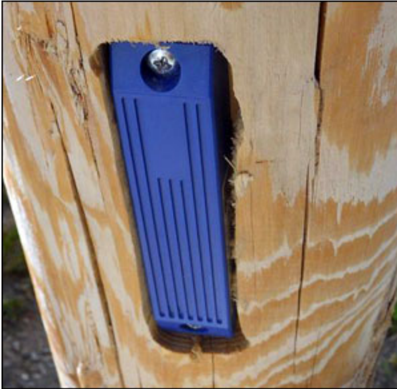
An Identec Solutions i-B2 RFID tag was screwed into a recess cut into each post.
