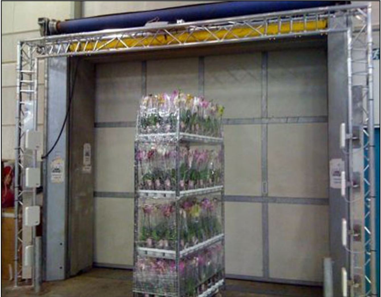
At Hamiplant's facility, an RFID portal installed at an outgoing dock door verifies that the trolley is loaded correctly.
