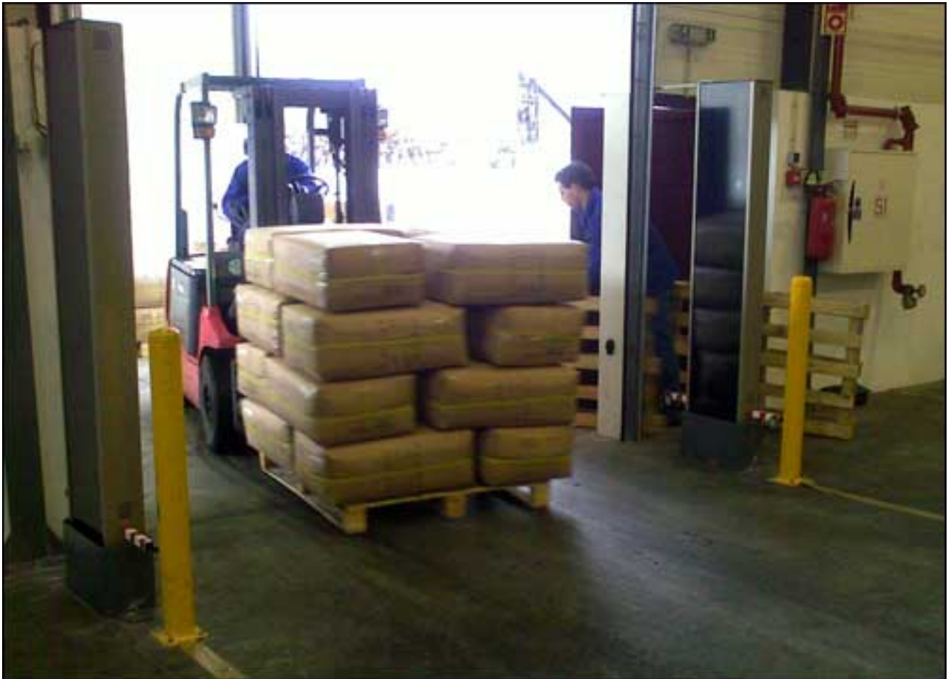
Warehouse employees bring RFID-tagged cases of material through a portal reader at the Marigold Industrial plant. The reader antennas are the black columns on either side of the door.
