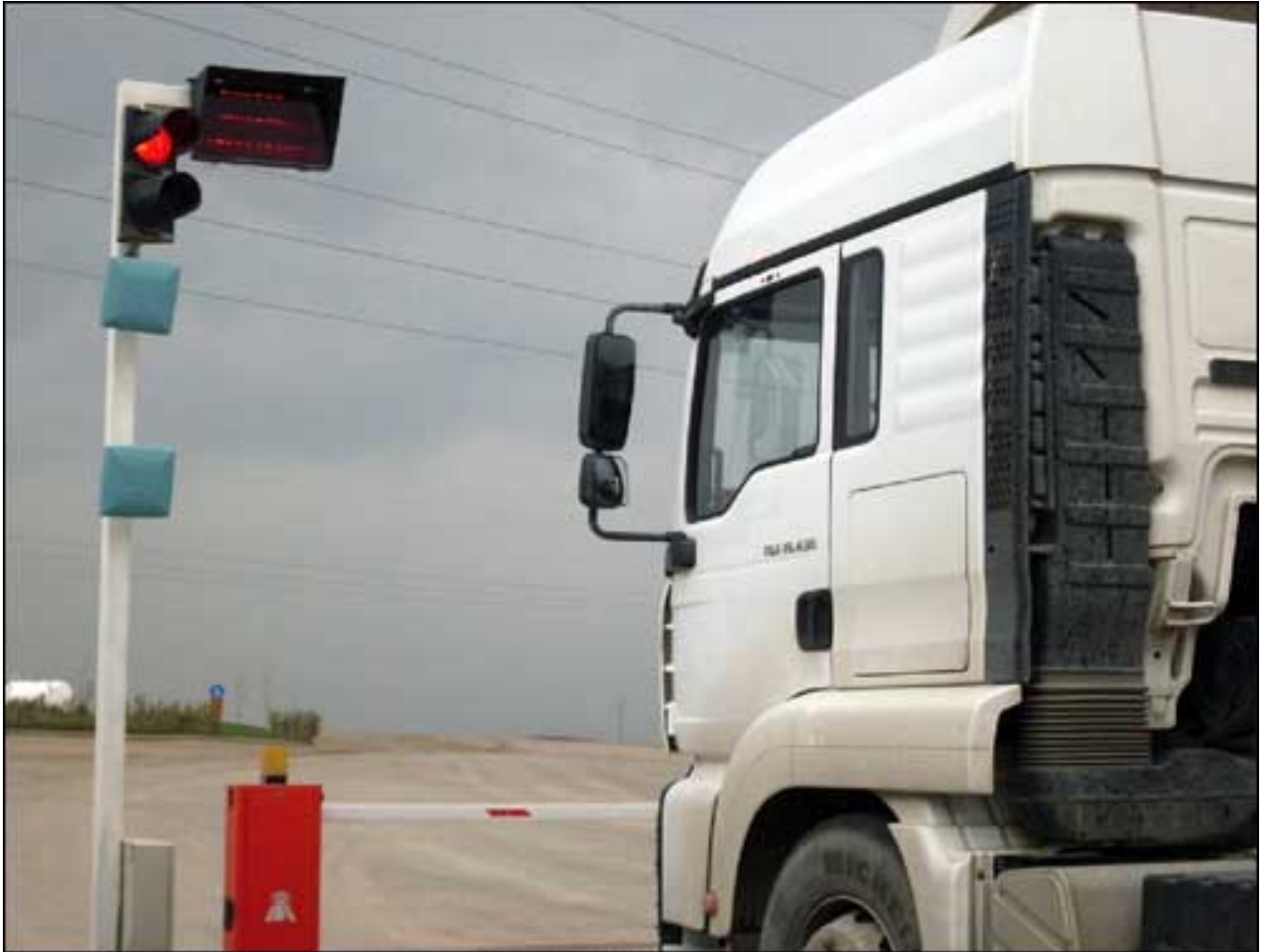
After the system identifies a truck, an LED panel instructs its driver to the proper loading bay.
