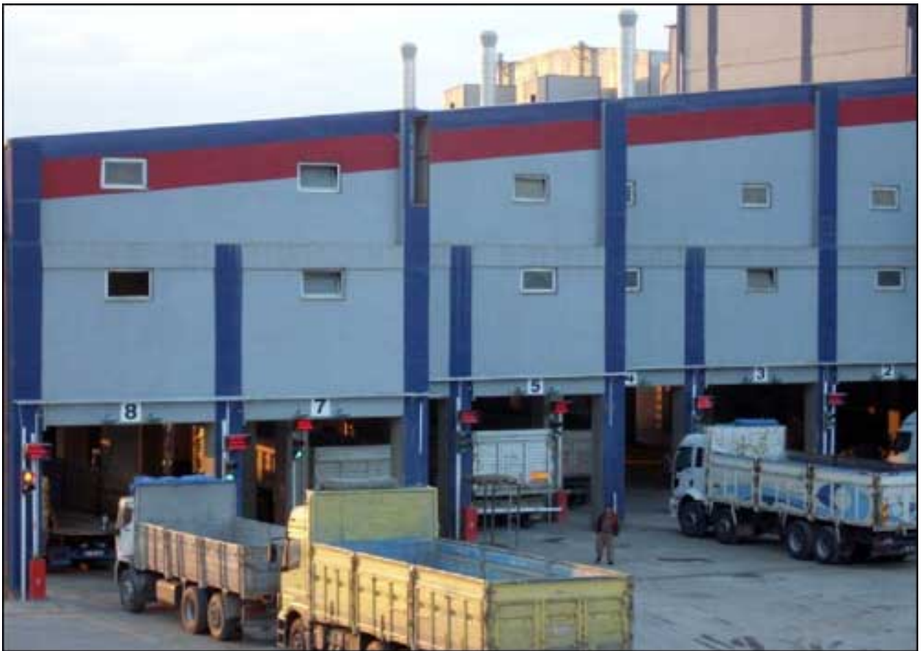
If a loading bay's RFID interrogator verifies an approaching truck is authorized to receive a load of cement, the gate raises automatically.
