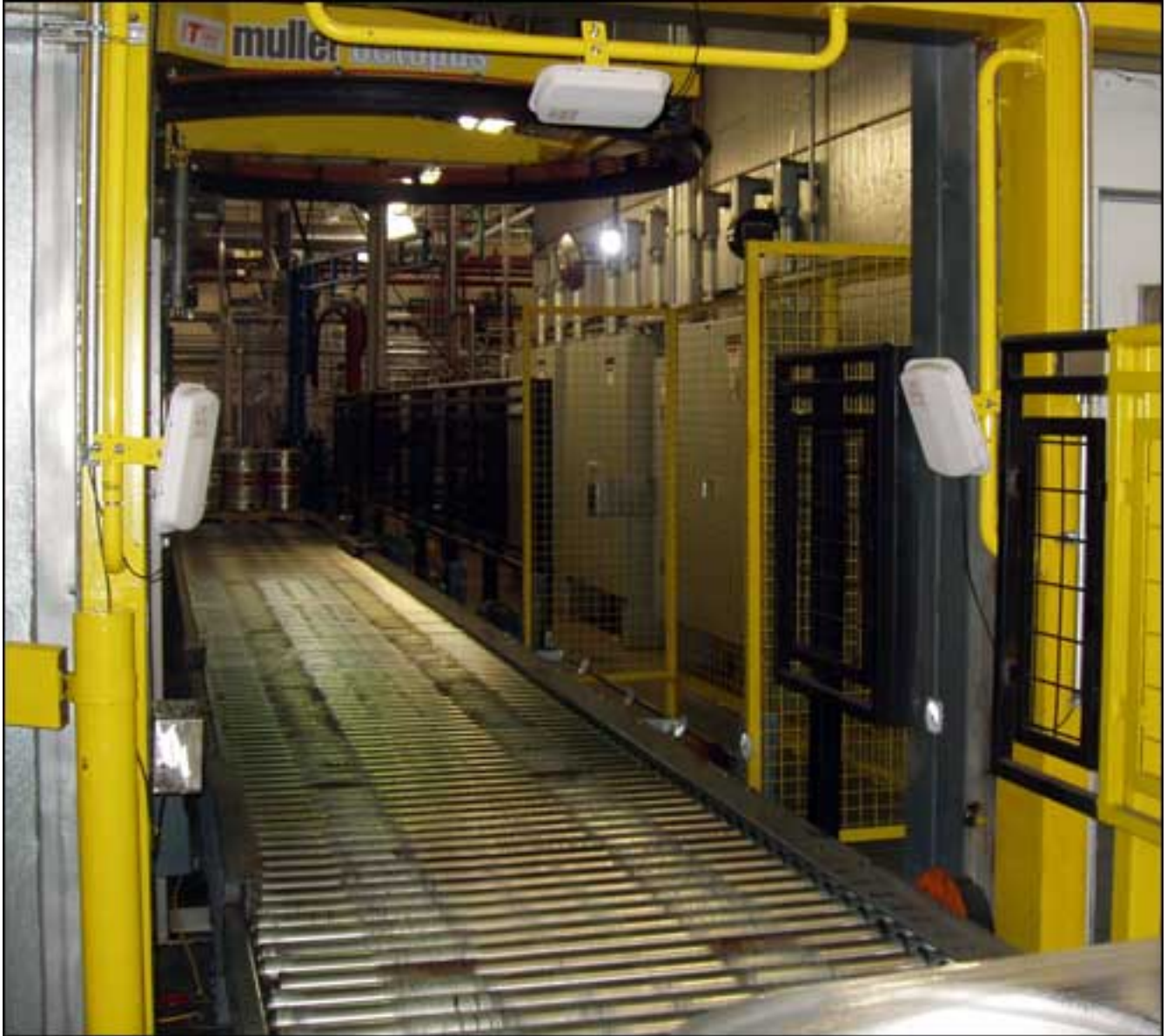
After a pallet of filled kegs is wrapped in plastic film, it passes through the fixed interrogator portal that reads the unique ID number encoded to each keg tag.
