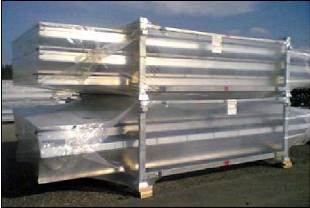
Tagged crates loaded with tagged facade elements.
