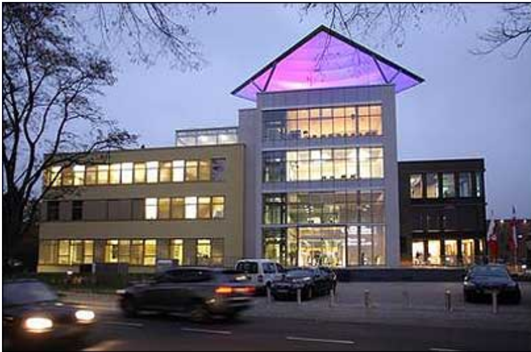
For the InHaus 2 project, the Fraunhofer Institute for Circuits and Systems is using a commercial building it has built to test the use of RFID on construction sites, and for energy-efficient building operations.
