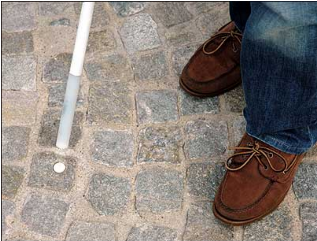
An antenna in the cane's tip reads the pathway's embedded transponders.
