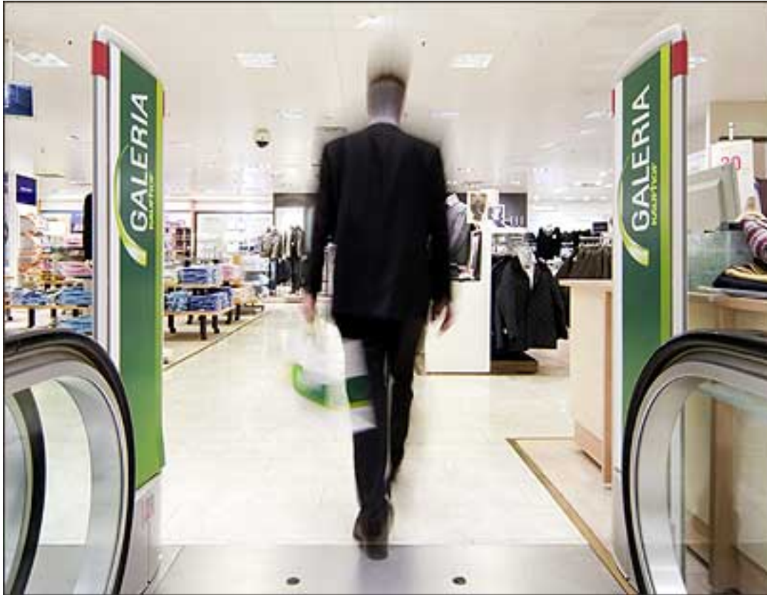
EAS/RFID antennas provide security monitoring at entrances, exits and fitting room areas.
